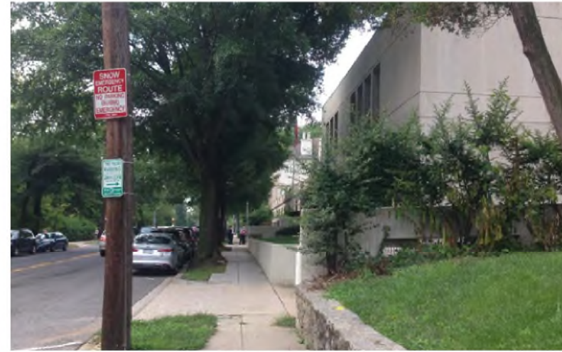
Fig. A-1.6.2 - Existing 34th Street frontage
