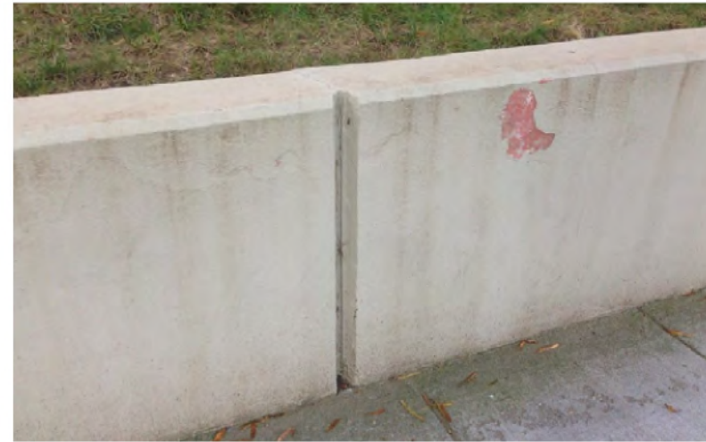
Fig. A-1.6.4 - Retaining walls along 34th Street.
