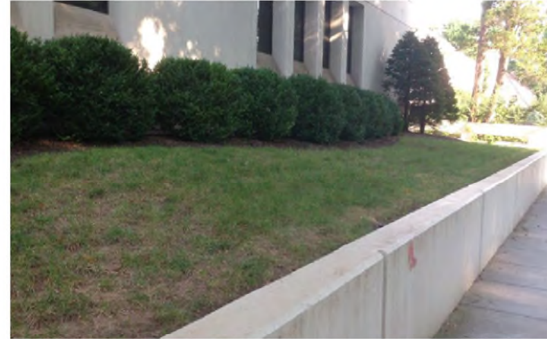
Fig A-1.6.3 - Retaining walls along 34th Street.
